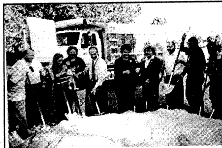
Commissioner Sosa and Neighbors start the work on 13th St.
